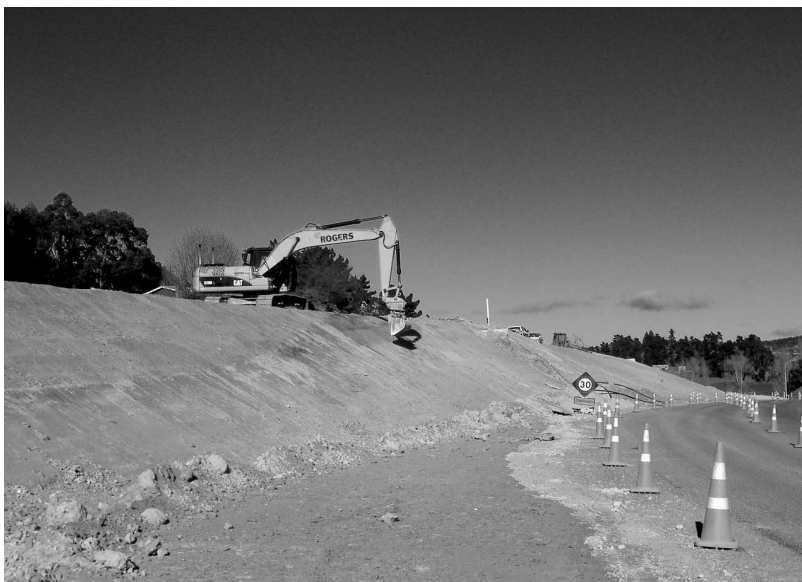
Batter trimming Apple Valley East intersection
