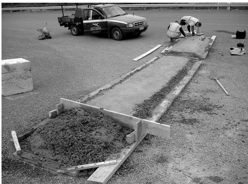
Construction traffic island Dominion Road
