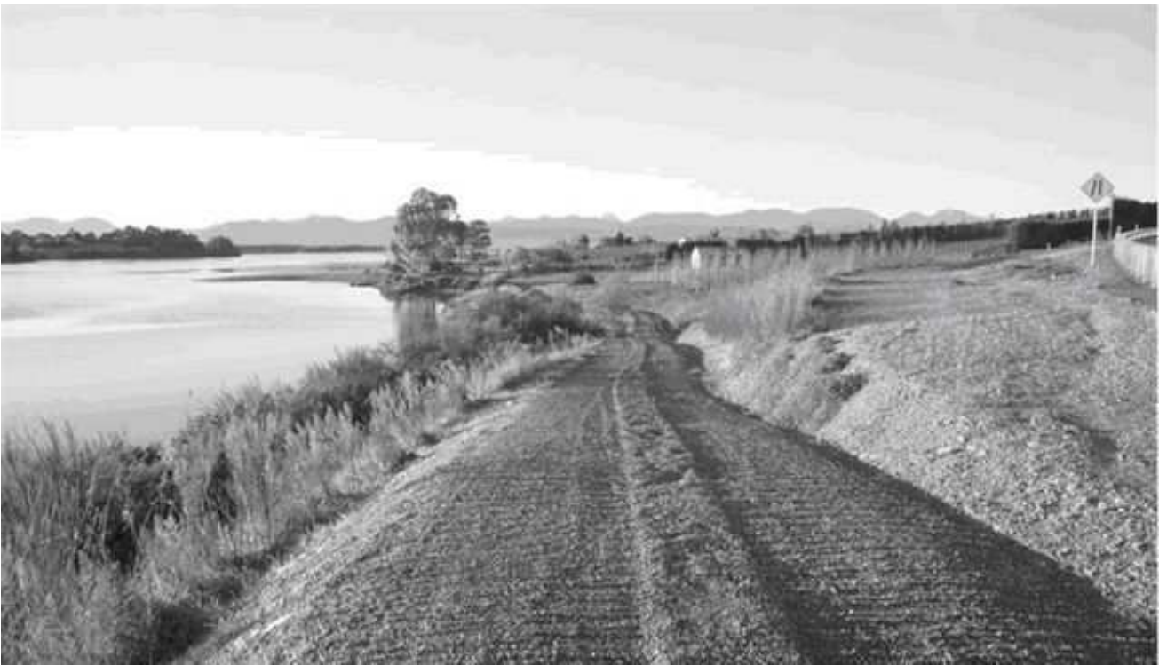
The new council-built walkway near Apple Valley Road. Critics say that it looks more like a road than a path and that it is too close to the estuary edge.
