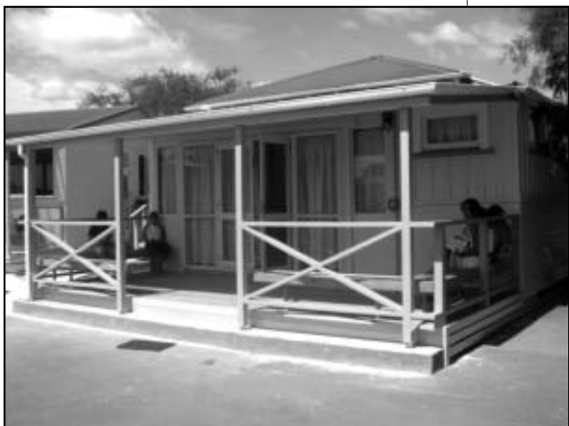
Mapua School's new library deck
