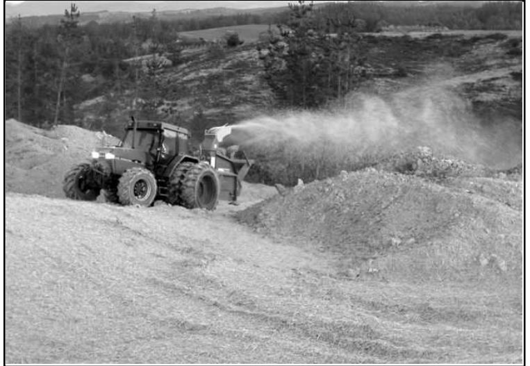
Spreading straw mulching to control erosion in the Chaytor Road area.
