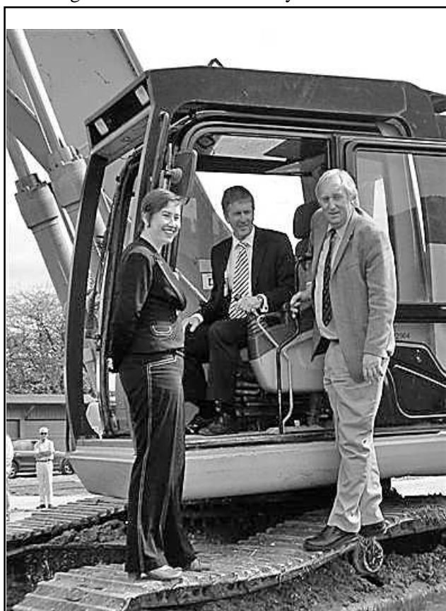
Deborah Hume, Regional Director of the NZ Transport Agency, on the excavator with Damien O'Connor at the controls, and Trevor Norris.
